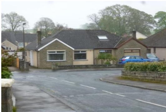
Photo 17. Bungalows on Manor Road
