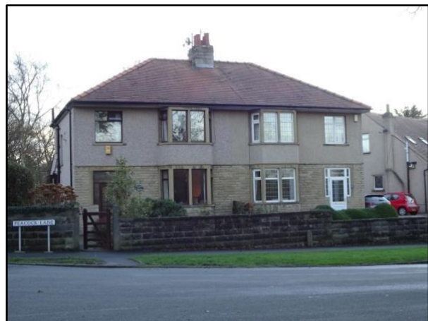
Photo 14. Semi-detached houses on Peacock Lane
