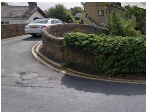
Photo 33. Canal Bridge on Hest Bank Lane
