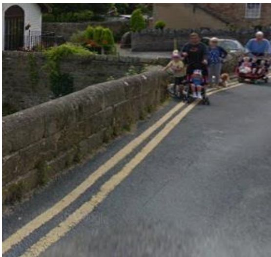
Photo 37. Pedestrians on Hest Bank Lane Canal Bridge
