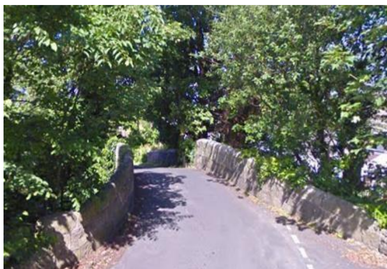
Photo 34. Canal Bridge on Hatlex
