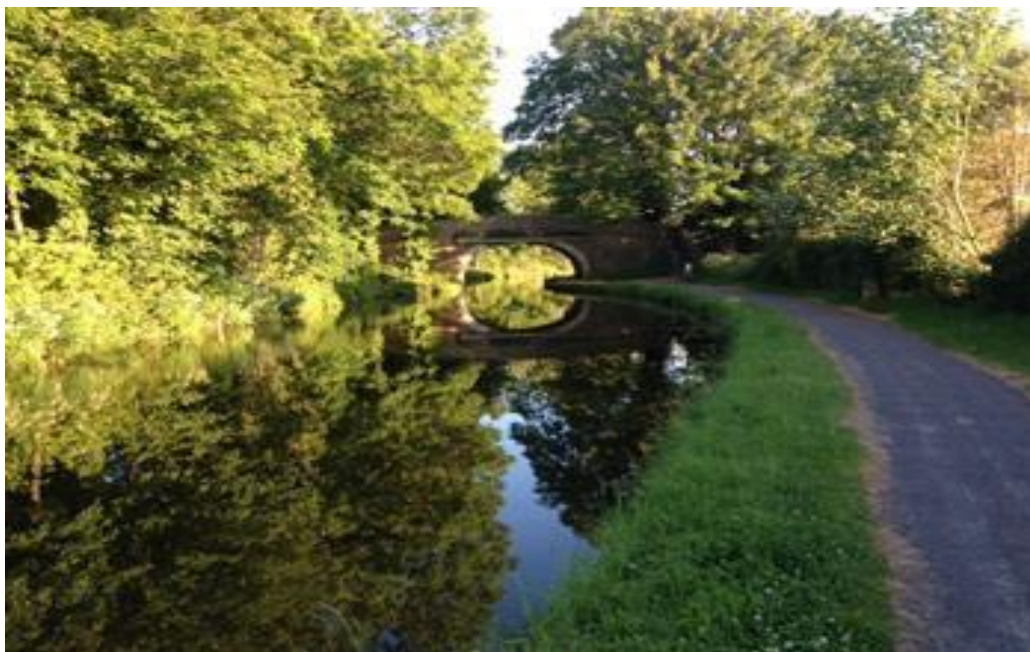
Photo 4. Hatlex Bridge (No. 119) on Lancaster Canal
